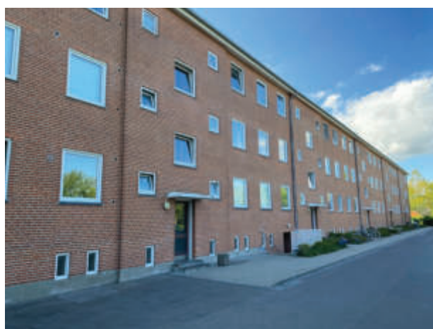
Facade Blok A
